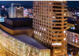
Performance Place Mixed-Use High Rise Facility
